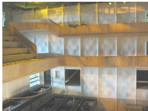
Figure 13. View of irregular plastered-wall before wooden laths are placed
