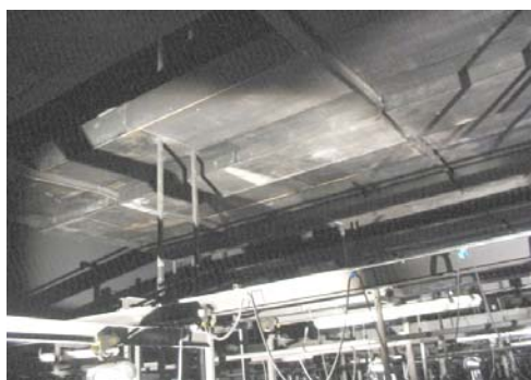
Figure 5. View on bridge level towards lowered ceiling and technical equipment
