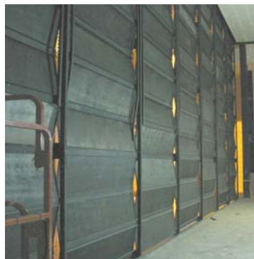
Figure 11. View from behind to the movable backstage wall with tilted wooden paneling
