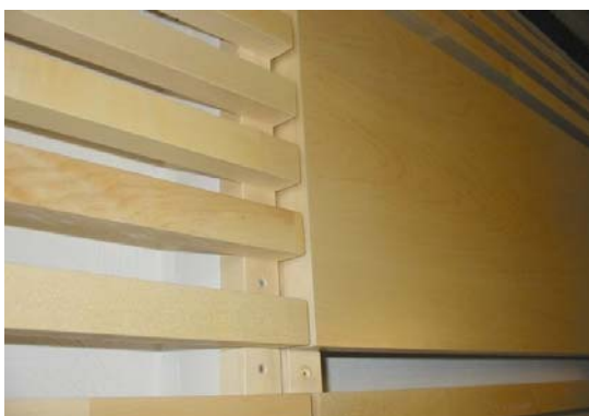
Figure 14. View of wall detail with wooden laths and closed panel
